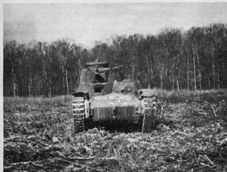
Jap medium tank 2597 head-on looks like U. S. General Grant with off-center turret. Gun shown is a low-velocity 57-mm. Hull is long, narrow and low. Light track (see below) has six medium bogie wheels.
